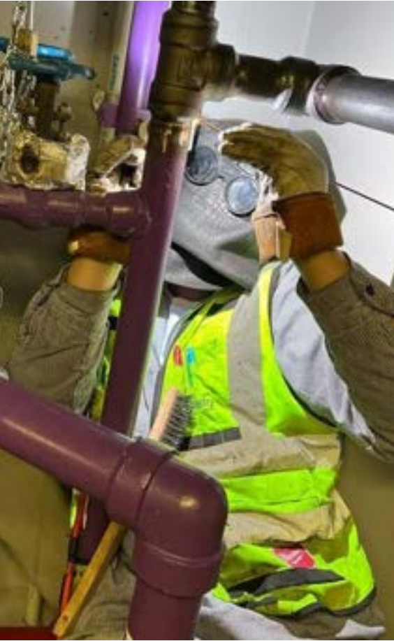
UA 32 member Damon Marr works on pipes.
