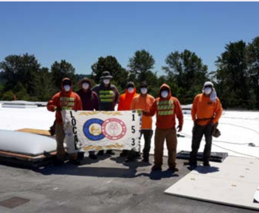
Local 153 roofers building a cool roof in Renton, WA.
