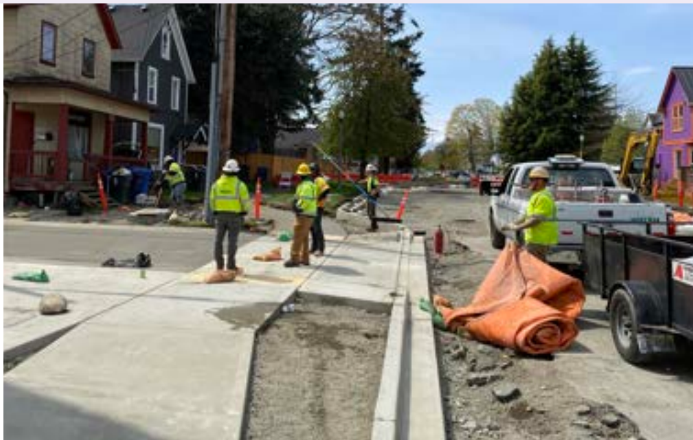
Laborers Local 252 workers installing a sidewalk.
