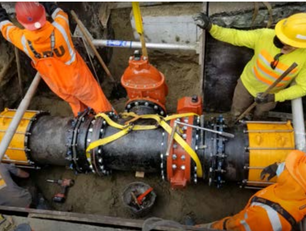
Plumbers and Pipefitters Local 32 water utility workers with Seattle Public Utilities installing a water main.
